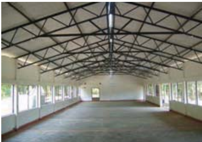
Dharma Salawa/Sunday School which is under construction in Giritale
