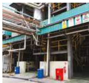
Safety signs in our manufacturing plants in Pasir Gudang, Malaysia
