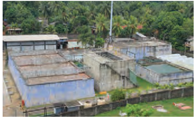
Waste water treatment plant at Biyagama, Sri Lanka
